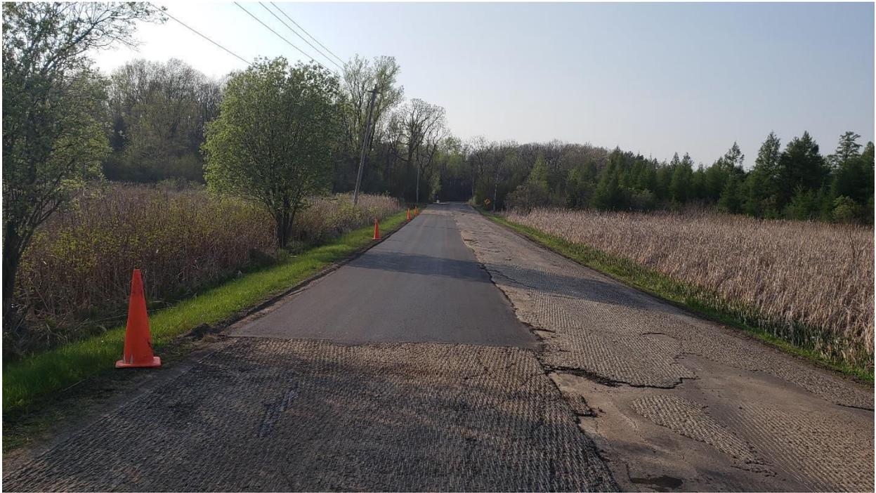
Unfortunately, there was another area that didn't look distressed until the loaded trucks drove over it which caused an emergency repair to be performed in order to keep paving as shown here.
